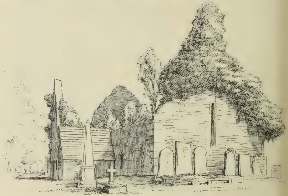
FIG. 1539.—Fetteresso Church. View from North-West.
